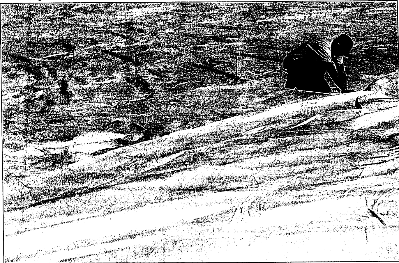
Harlin Andresen, an employee with the Cedar Rapids Recreation Department, smoothes out the seam of a giant plastic liner Wednesday afternoon in the parking lot of the Ellis Park pool. The 150-foot by 80-foot liner is used to line the ice rink at Bever Park. According to recreation facilities manager Dave Bowser, the liners must be repaired every year due to tears caused by ice skates.
